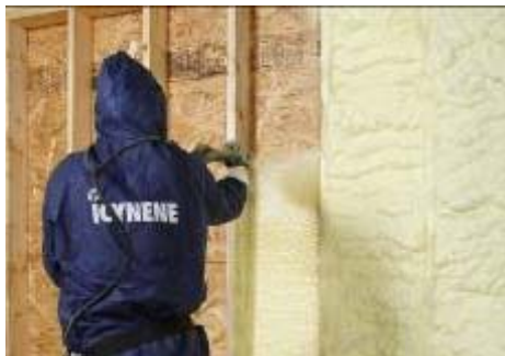
Icynene is installed in adherence with local building codes. Once applied, finished appearance may vary from photo shown.
